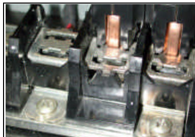
B. "Z" clip, clamped to . bussbar with 10-32 screw.
